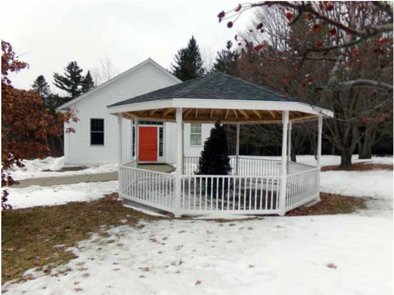
Richardson Gazebo constructed by RWRichardson Construction
